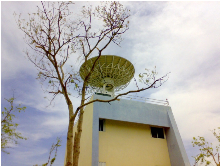
MODIS Direct-Broadcast X band systems Antena en ECOSUR - Chetumal, Q.R.
